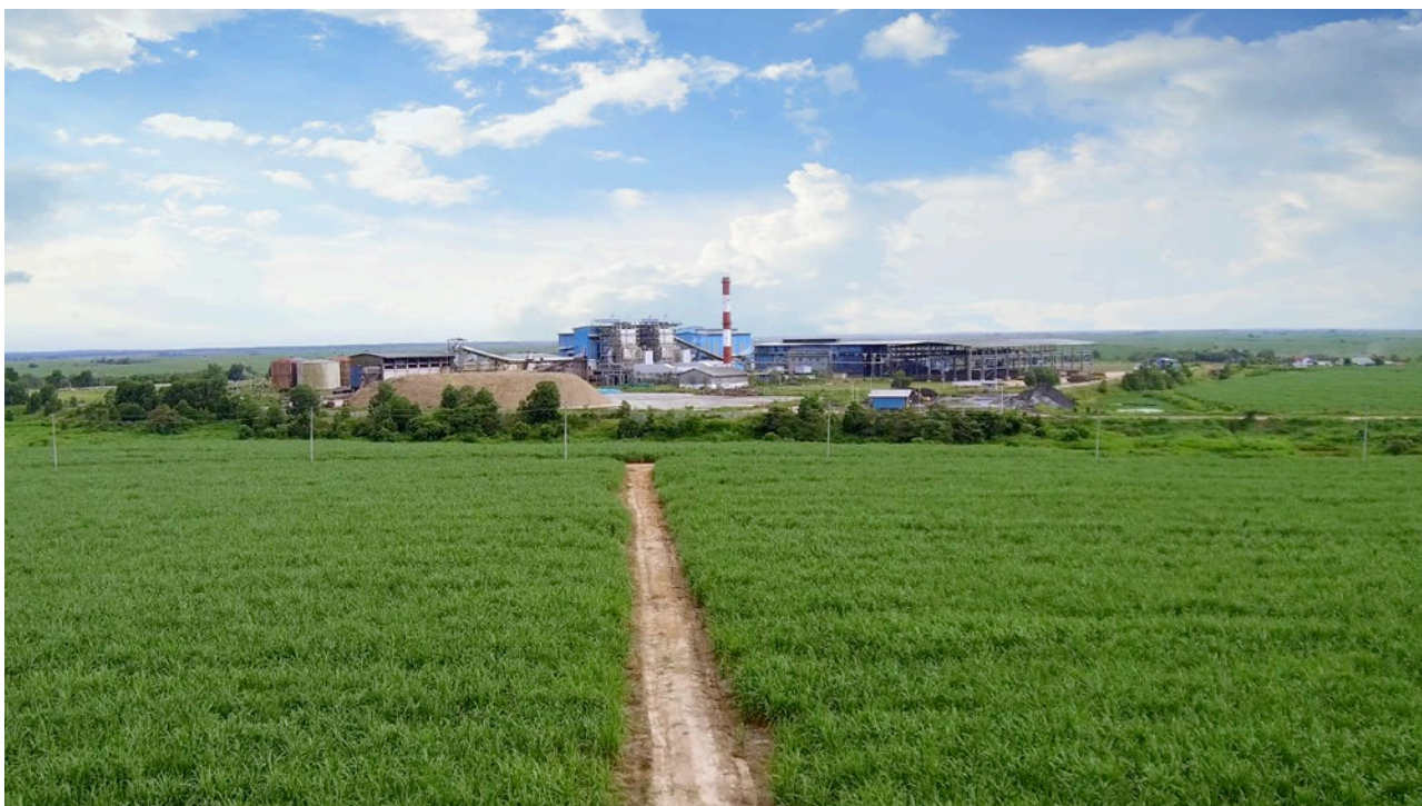
Integrated Sugar Cane Plantations and Sugar Production Facility at South Sumatra
